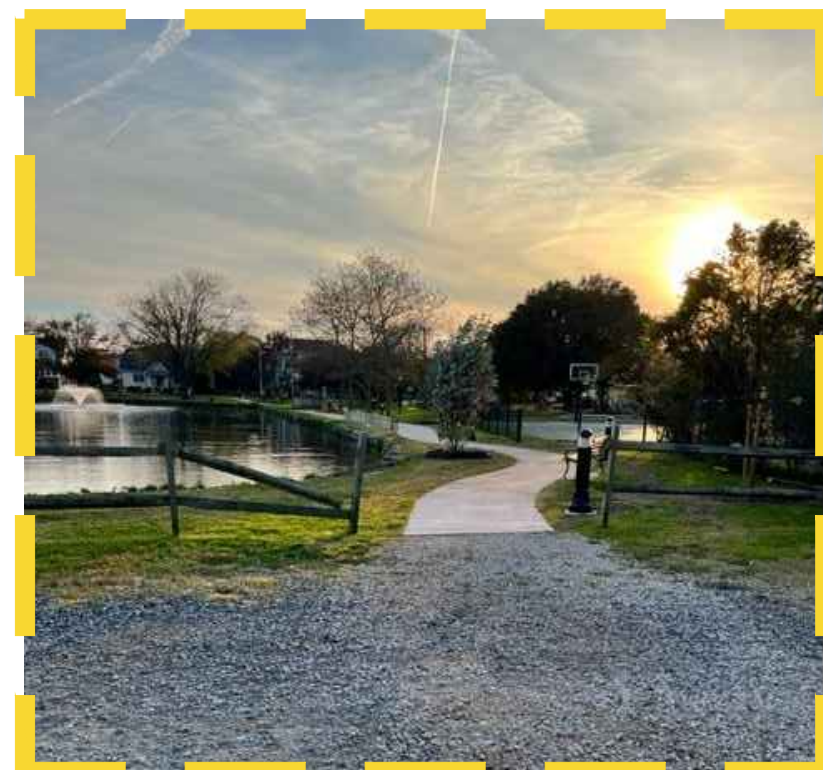
CONSTRUCT 5' SIDEWALK ALONG EAST SIDE OF GRAVEL DRIVE FROM KIWANIS PARK TO ADA ACCESSIBLE TENNIS COURTS
