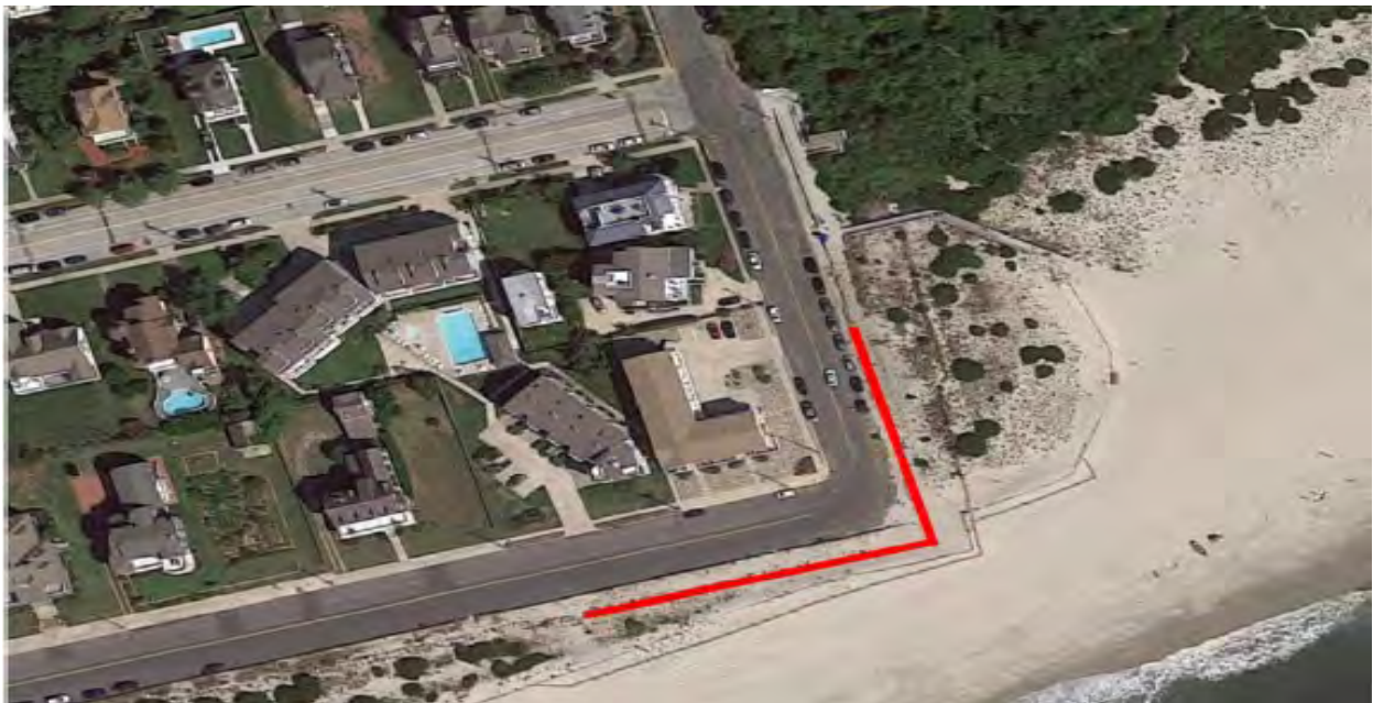
Figure 13: Superstorm Sandy Impact in Seawall Area
