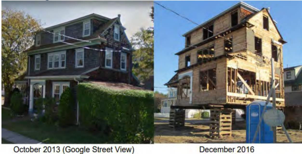
Figure 19: Recently Elevated Structure at the Corner of Kearney Avenue and Jefferson Street in Frog Hollow
