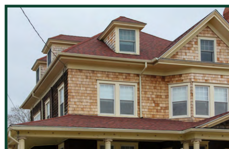
✓ Appropriate replacement of deteriorated elevations of shingles
