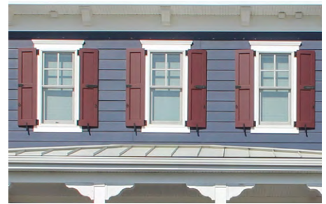
Double-hung window with operable shutters
