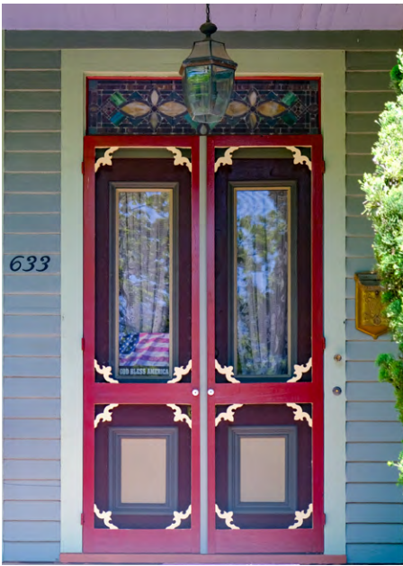
Screen door does not obscure primary door behind
