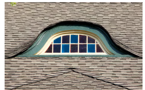
Colored glass lights in an eyebrow roof dormer
