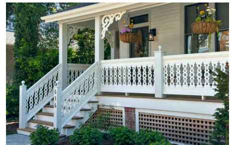
Porch with jig-saw cut balusters and latticework
