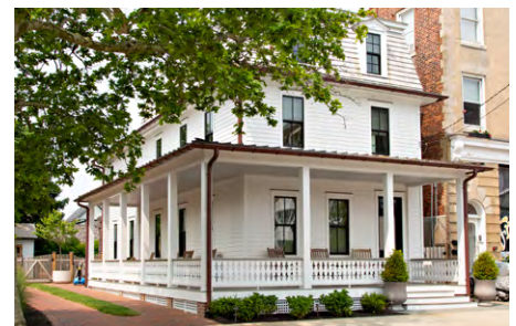
Minimally visible rear addition
