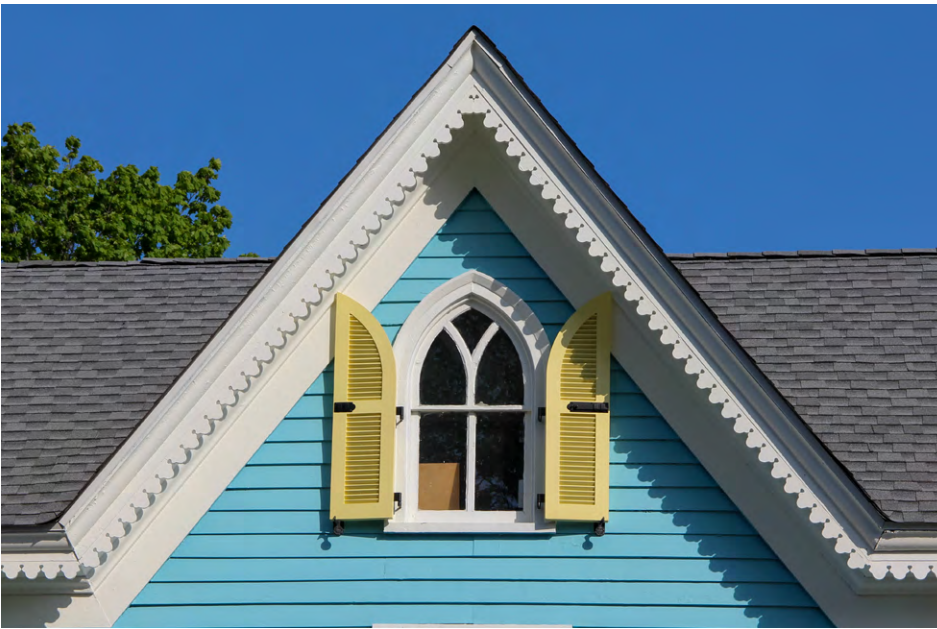
Gothic arched window with properly-sized functional shutters
