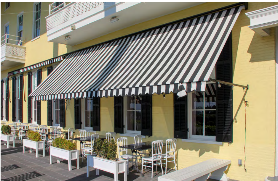
Striped canvas fabric awning with traditional operating mechanism
