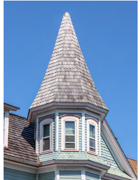
Cedar wood shingle roof
