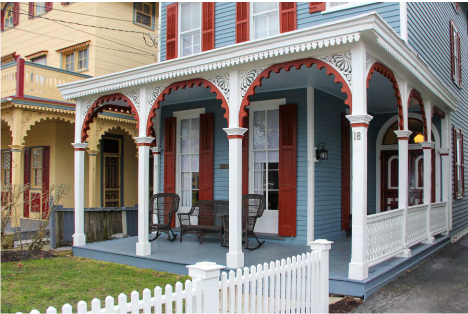
Elaborate jigsaw-cut porch arches
