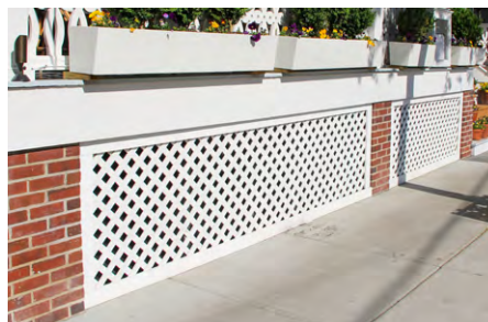
Foundation piers should always be infilled with framed latticework
