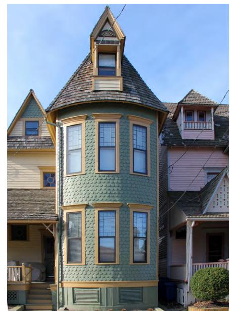
Patterned shingles on a round tower of a Queen Anne style house
