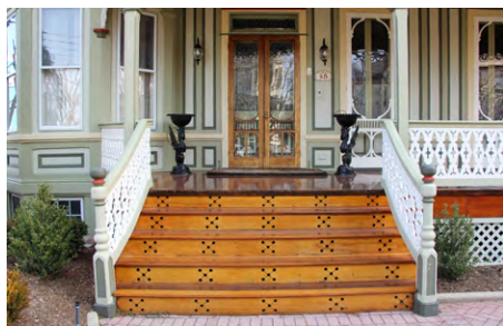
Wood stairs with embellished risers
