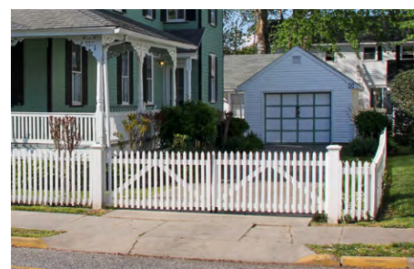
Hinged driveway gate
