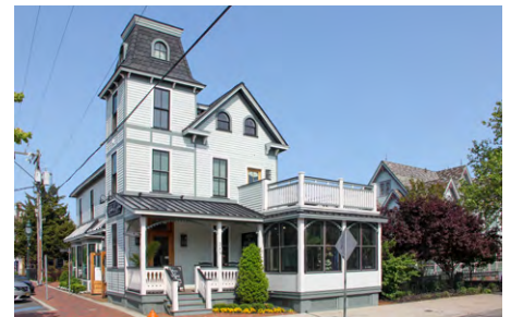
Tower addition based on documentary historical evidence
