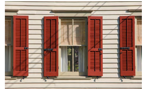
Louvered panel shutters on a Colonial Revival style house
