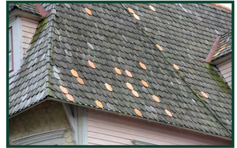
✓ Appropriate selective replacement of extensively-deteriorated elements
