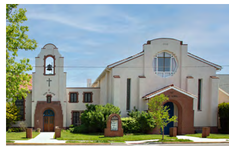
Cape Island Baptist Church, 115 Gurney Street
