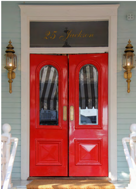
Pair with arched glazing and rectangular transom above
