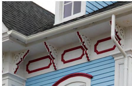
Bracketed cornice eaves
