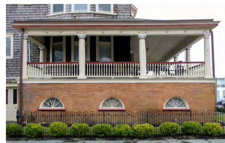
Yellow brick masonry foundation with semi-circulate windows
