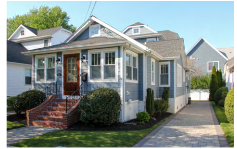
Rear addition with similar roof pitch and exterior cladding materials
