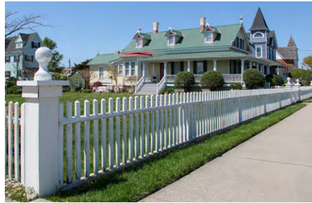
Wood picket fence with corner post
