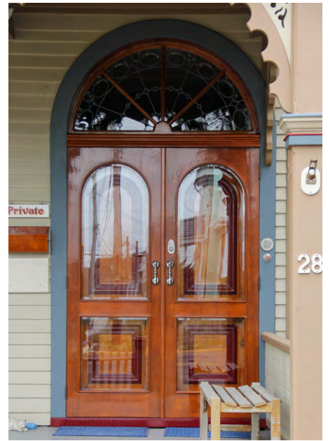
Storm door glazing follow similar pattern to primary door behind
