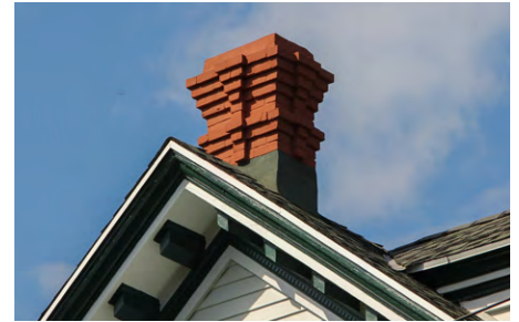
Decorative masonry chimney
