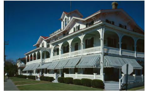
The Chalfonte Hotel | 301 Howard Street
