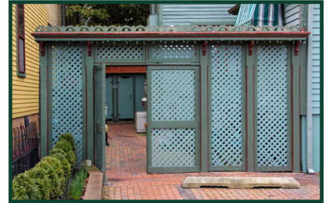
✓ Appropriate screening of mechanical equipment and rubbish
